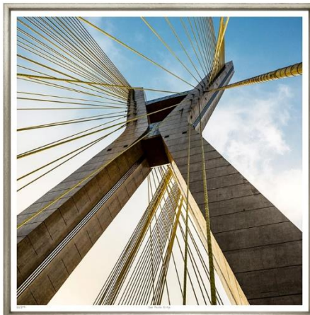
TS2397 | Sao Paulo Bridge
