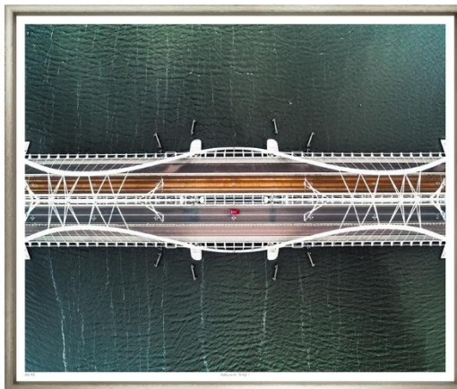
TL2176 | Netherlands Bridge
